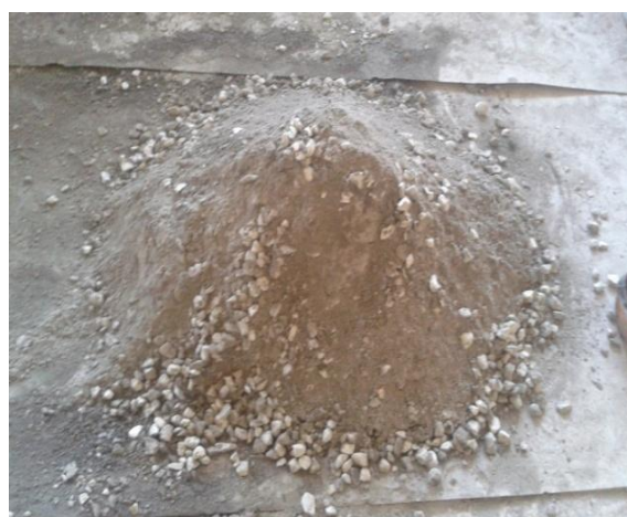
Fig. 2. Mixing of ingredients for making concrete.
